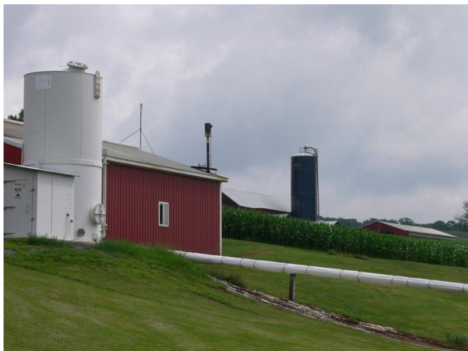
Fig. 23: Manure is pumped to the digester at Twin Birch Farm in Skaneateles, New York.
