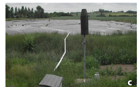
Figure 1. Types of anaerobic digesters: a) plug-flow b) complete mixed, and c) covered lagoon
