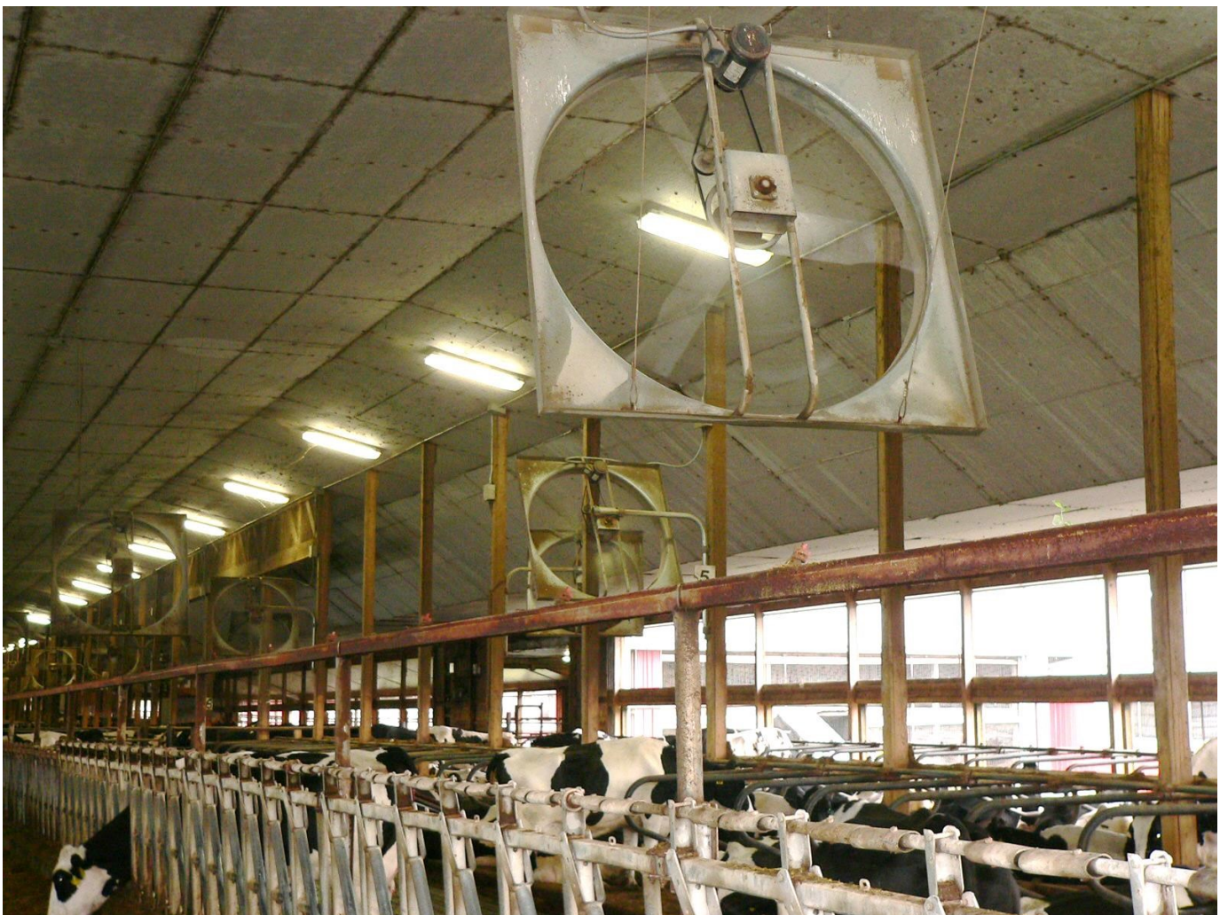
Figure 18. Cows in this freestall barn in New York are kept cool in the summer with large fans and side curtains that open and close depending on the temperature. Photo: Carolyn Betz
